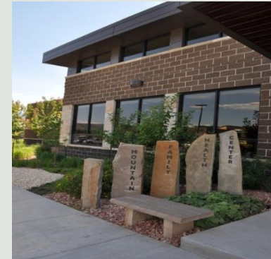
Mountain Family Health Centers, Glenwood Springs
