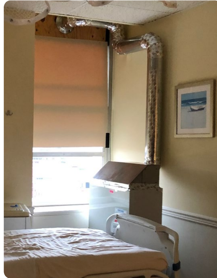
Negative air machine ducted out the window
