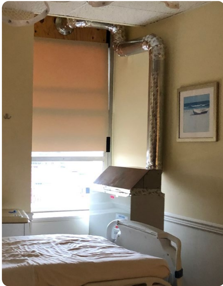
Negative air machine ducted out the window
