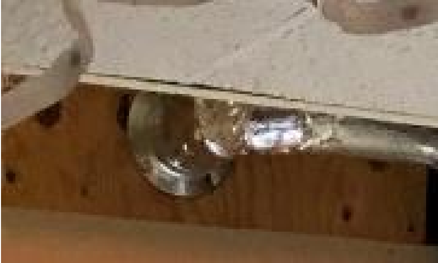
AIR EXHAUSTED THROUGH WINDOW VIA DUCTWORK FIT THROUGH PLYWOOD
