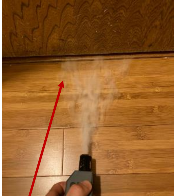
Smoke test: Use non-toxic smoke to see if it gets sucked into the room
